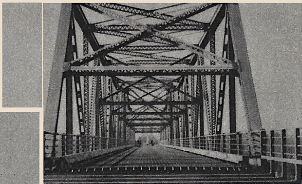
Above—View of one of the bridge's continuous truss sections.
